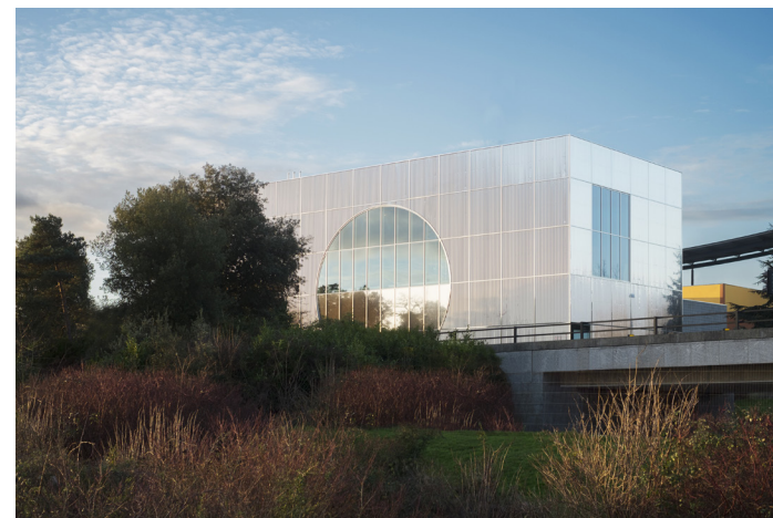
Photo: 6a architects
